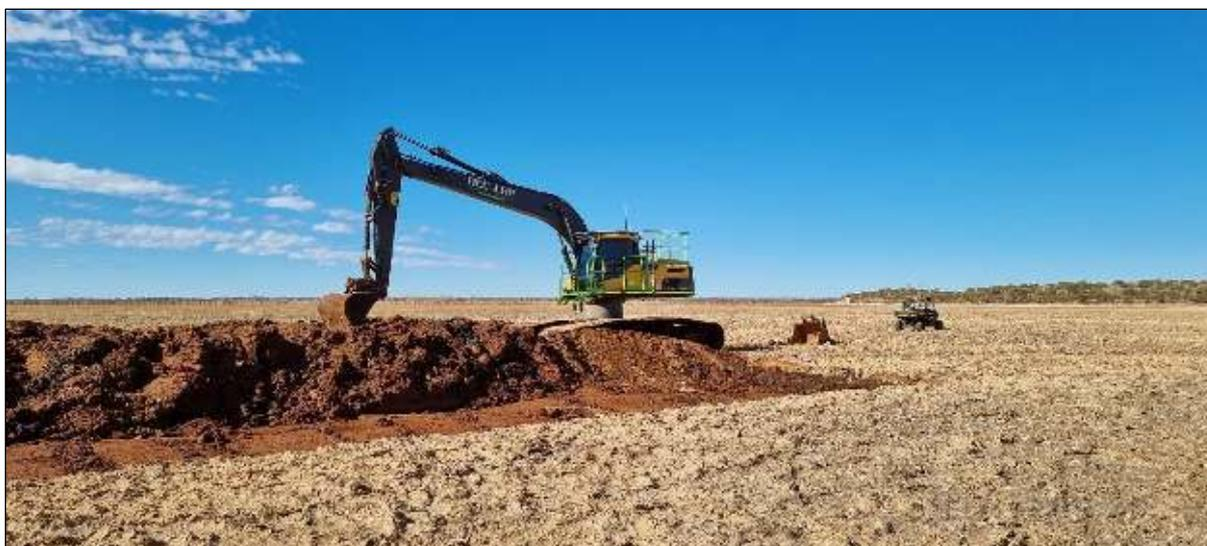
Figure 2: Establishing causeways for 2022 drilling campaign
